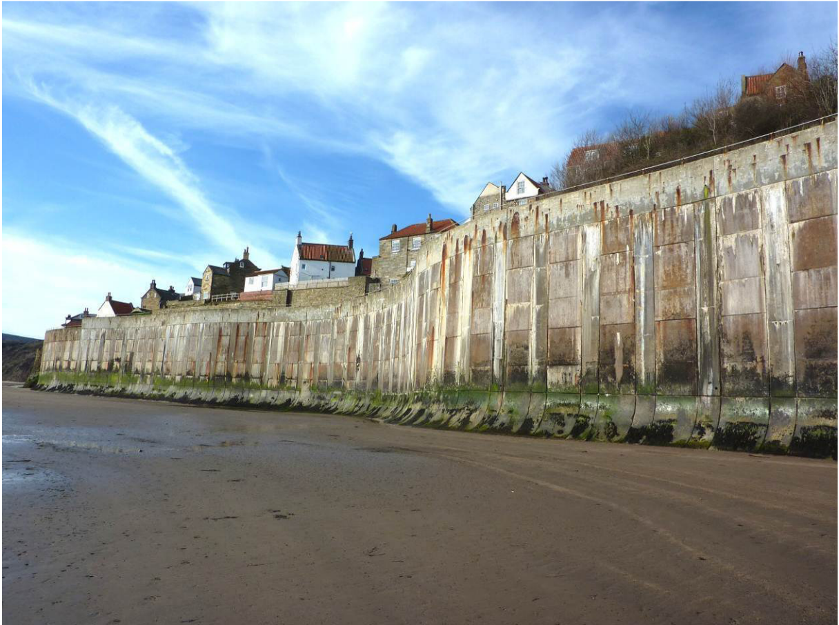
Figure 2.3: View looking south along concrete sea wall
