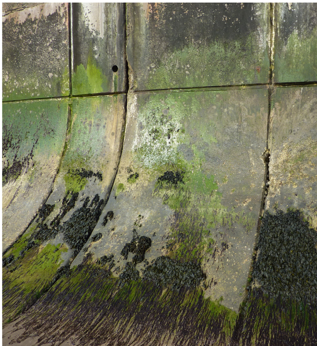
Detail of toe of concrete sea wall showing extensive loss of joint material and loss of concrete surface
