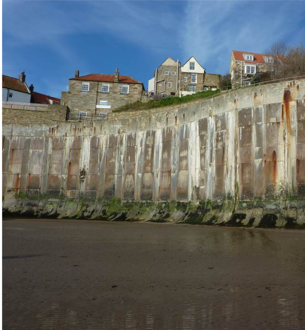
Detail of toe of concrete sea wall showing extensive loss of joint material and loss of concrete surface
